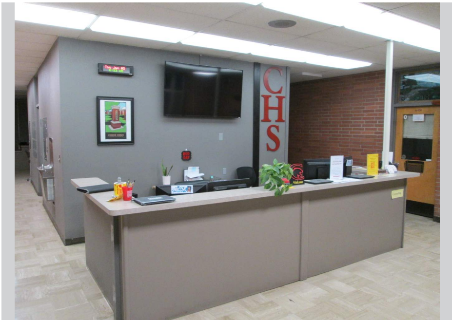
ADA accessibility counter height at reception desk required
