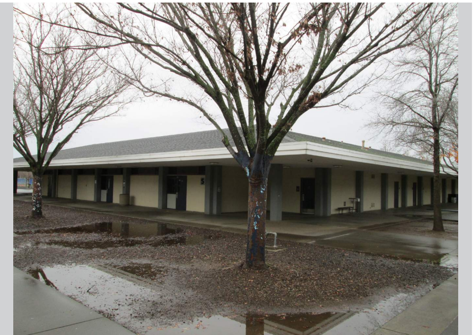
Exterior drainage improvements required to prevent puddling
